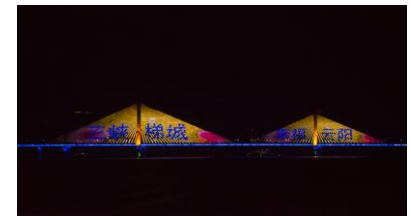
An Illuminated Bridge on the Yangtze River
