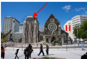
Christchurch Cathedral which lost the steeple (arrow) in the foreground and our hotel (H), undamaged in Cathedral Square.
